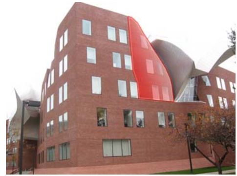
Figure 1.0 Complex-curved masonry construction PROJECT: Case Western Reserve University LOCATION: Cleveland, Ohio ARCHITECT: Gehry Partners
