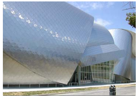
Figure 2.5 2D fabrication for 3D application 2D fabrication of metal to produce 3D form
