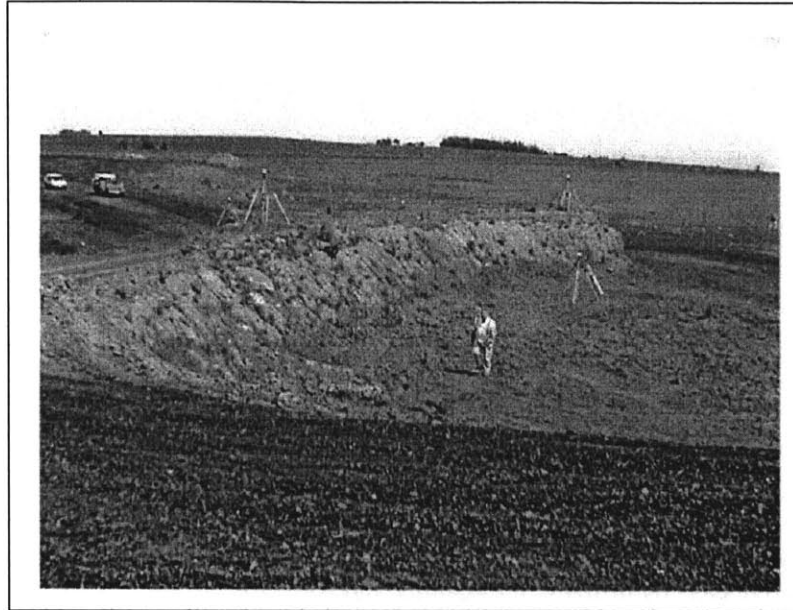
Figure 2.15: Photograph of stockpile used in Iowa DOT pilot experiment
