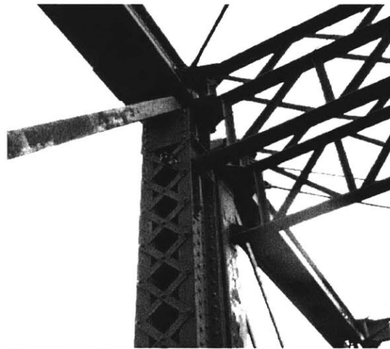
Figure 45: Connection on Old Northern Avenue Bridge
