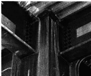
Figure 16: Example of Moment Connection Courtesy of University of Wyoming [18]
