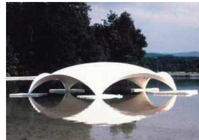
An image of a scaled model of a thin concrete shell by Heinz Isler from the exhibition "The Art of Swiss Engineering" 2005 Image: Heinz Isler http://web.mit.edu/museum/exhibitions/galleries/swisslegacy/1.html
