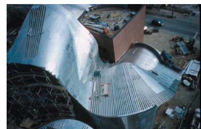
Developable surface in Gehry's architecture. It is clearly visible how the geometric constraint of straight lines of ruling is directly linked to the construction constraint.
