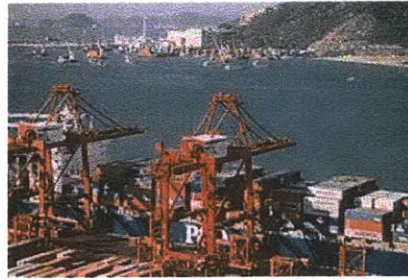
Figure 23. RFID readers would be scattered throughout a port and on cranes in order to have a constant flow of information with total coverage. The signals would be transmitted to the central data center via Wi-Fi/Wi-Max technology. Photo Source: http://128.121.48.70/images/guides/hongkong/travel/customs1.jpg
