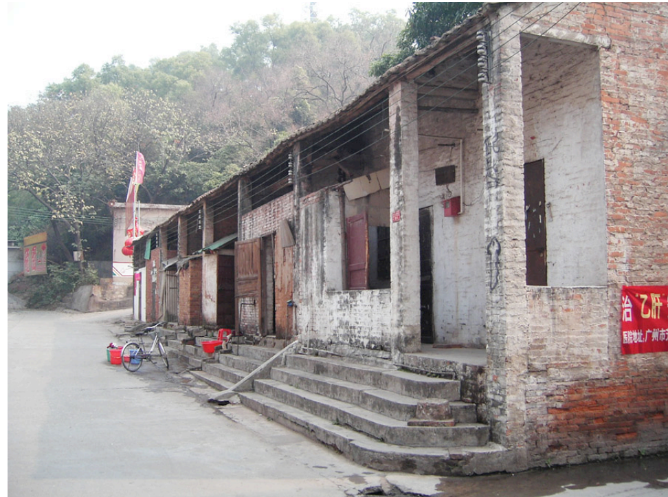
Figure 3.17. Temporary Housing in Gaoming, off Canjiang Road. Source: Field Research, January 2005.
