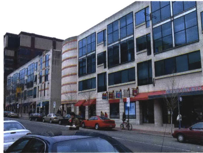
FIGURE 39: 3401 WALNUT STREET, CA. 2005
