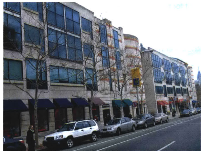
FIGURE 40: 3401 WALNUT STREET, CA. 2005
