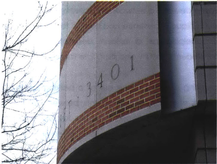
FIGURE 37: 3401 WALNUT STREET, CA. 2005
