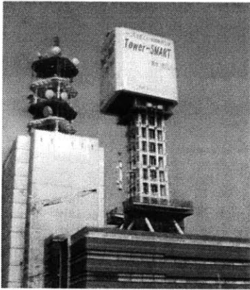
Figure 18 - Tower-SMART building system - Shimizu Corporation, Japan
