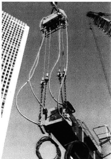
Figure 45 - Components of Mighty Shackle Ace - Shimizu Corporation, Japan
