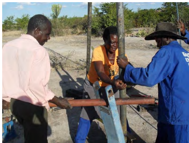
Photograph 51: Villagers involved in borehole rehabilitation (Source: ZWP, 2012)
