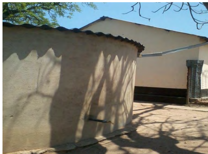
Photograph 45: A water harvesting tank at Mbilashaba School
