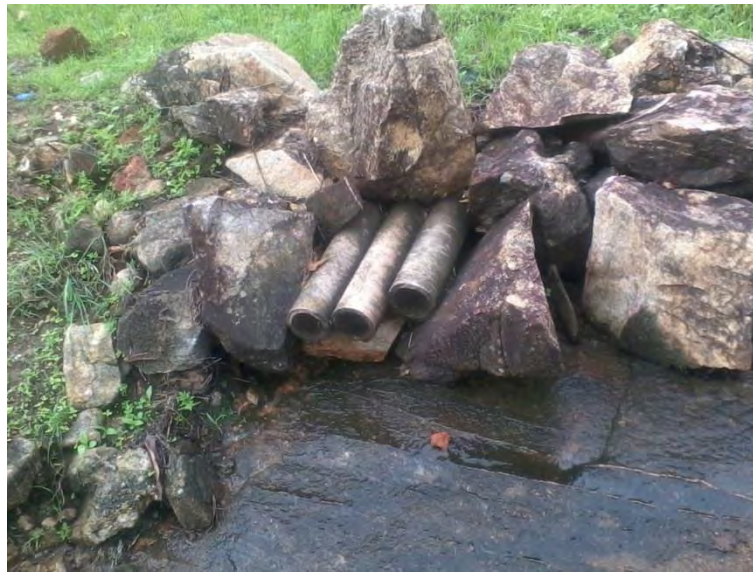
Photograph 23: Spreading water - pipes that harvest water from the rock outcrop and drain it into the 'immigration centre'
