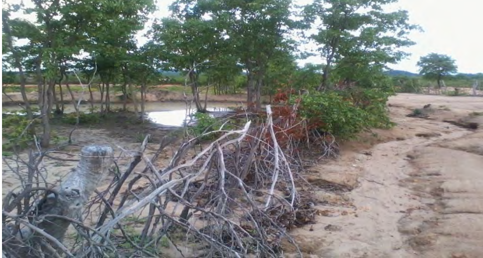
Photograph 58: Small dam (product of 'erosion-killing')
