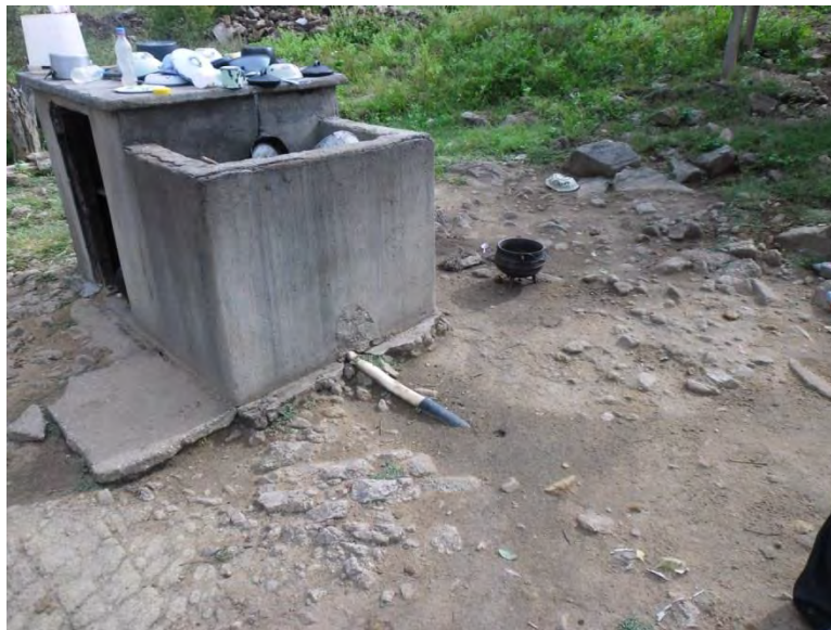
Photograph 25: Sinking water - dishwater is drained into an underground tank, the 'social tank' through the white and black pipe at the base of the trough
