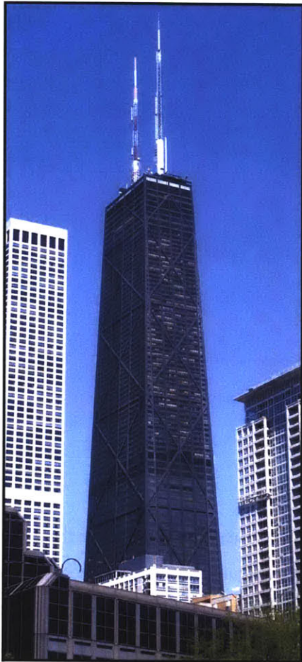
Figure 4 - 2: John Hancock Center (Chicago) [2]
