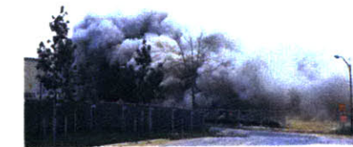
implosion of outmoded hospital
