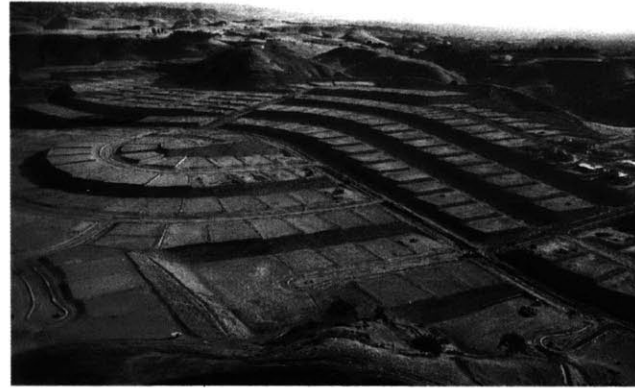
hillside terraced for subdivision construction!
