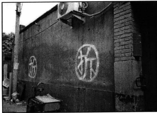
Figure 12. The Chinese character for demolition, “chai,” painted on the wall of a courtyard home.
