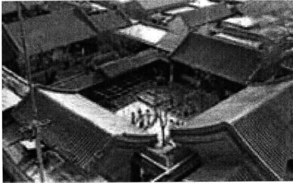
Figure 3. A classic courtyard house.
