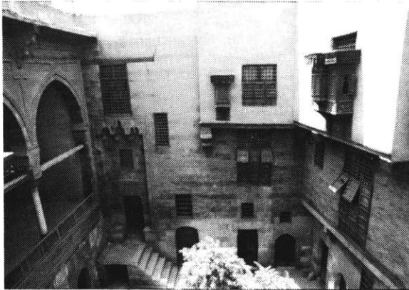
Maq'ad in the context of a traditional house
