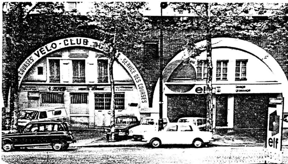
fig.3 The framework of the Parisian viaduct
