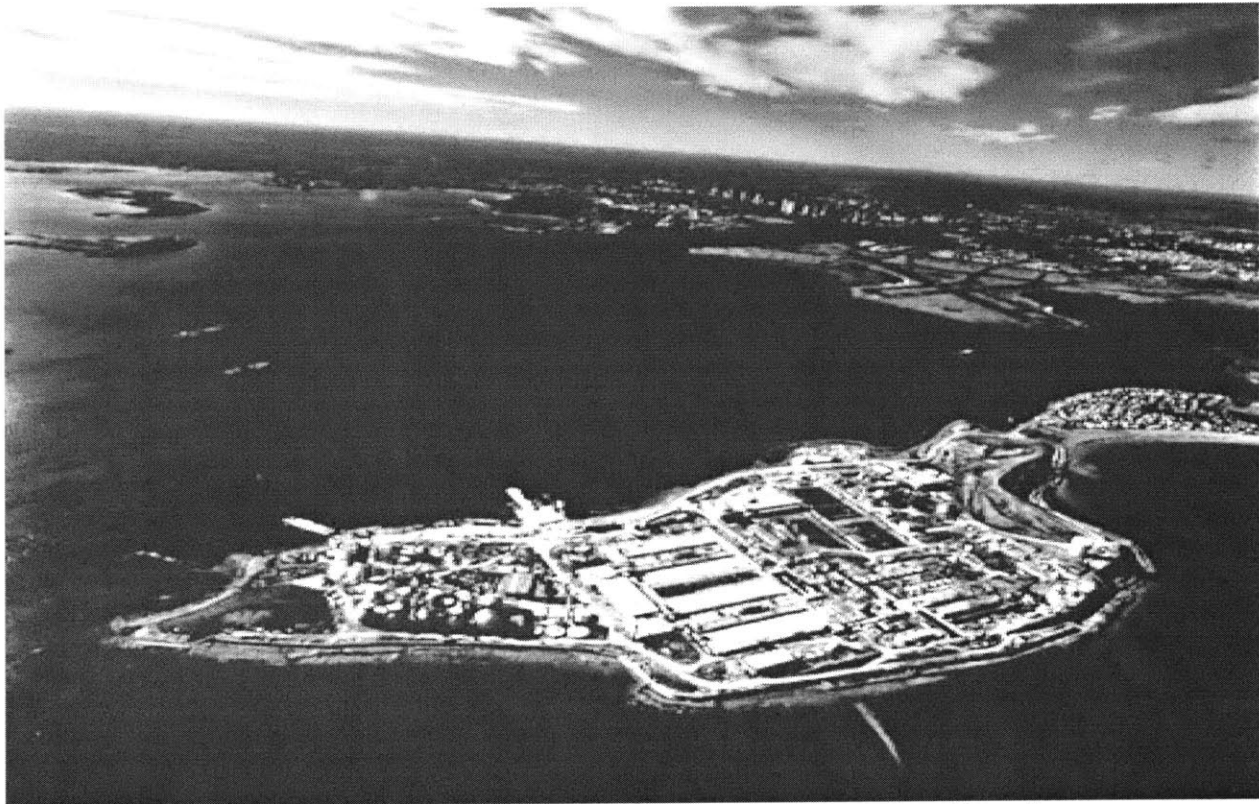
Figure 5-1: Boston Deer Island Wastewater treatment plant ( http://www.bryant-engrs.com/projects/deer.htm )
