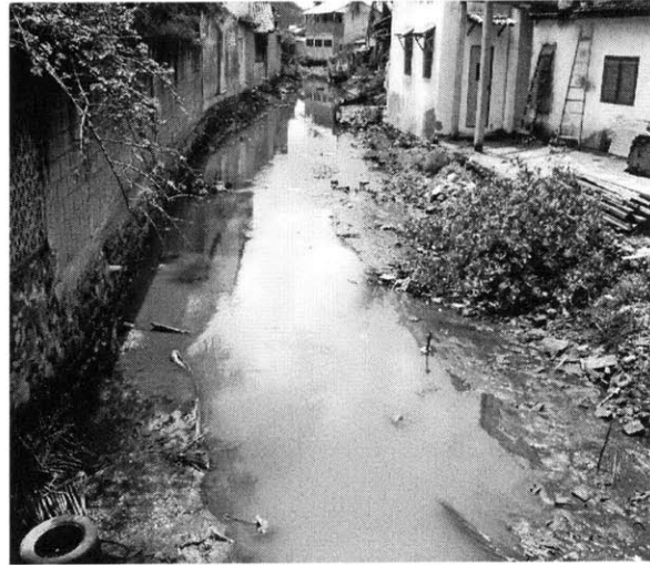
Figure 1.12: River of sewage
