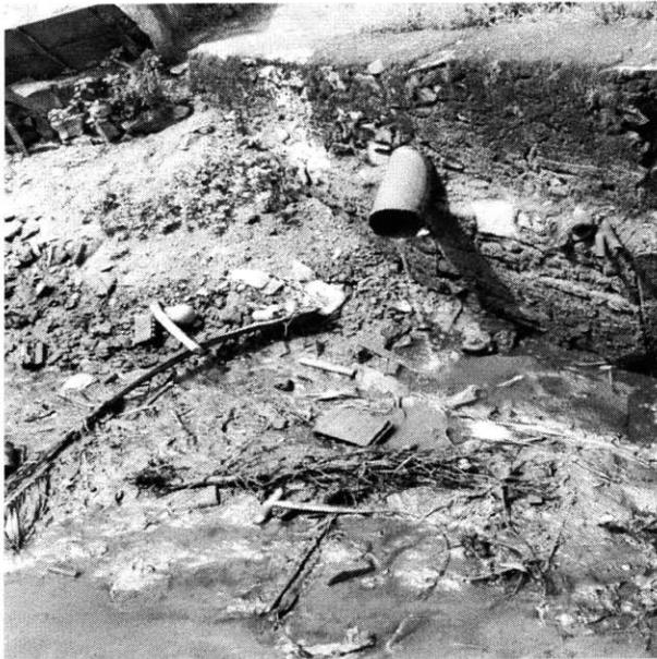
Figure 1.7: Sewage Discharge into Street (2)
