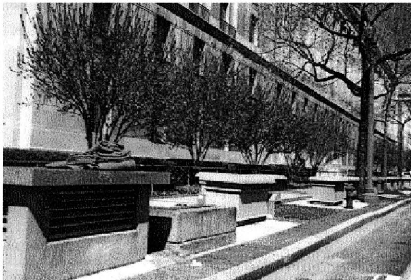
Figure 15: Landscaping used to protect building's facade.
