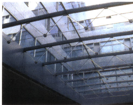
Figure 28: Zwitserleven glass and steel truss system [30]
