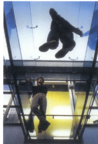
Figure 22: a) Loading test on completed bridge using employees from Kraayvanger Urbis, b) Looking upward into completed footbridge [38]
