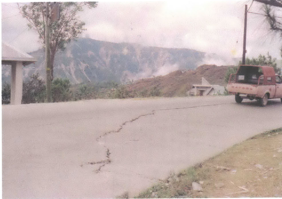
Figure 3.14 Effects of the 16 July 1990 Earthquake (Geotecnica, 1990)
