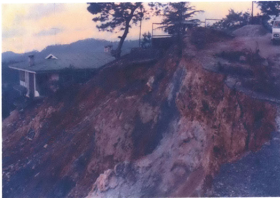
Figure 3.9 The Crest of the Landslide (Geotecnica, 1987)
