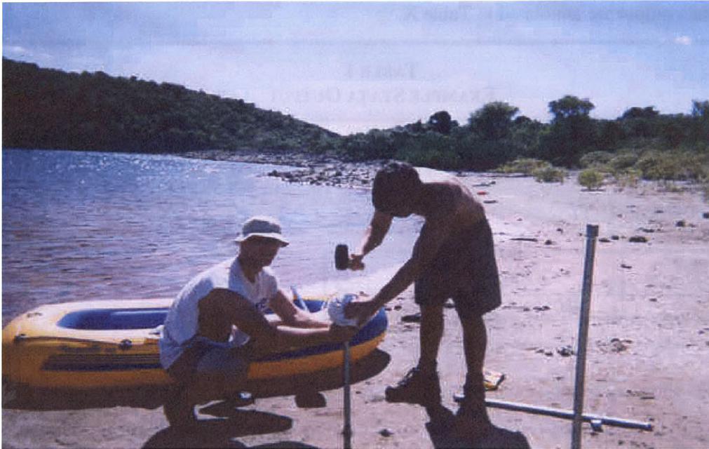
FIGURE 15 INSTALLATION OF MINI-PIEZOMETERS (Southside Pond, St. John, USVI)
