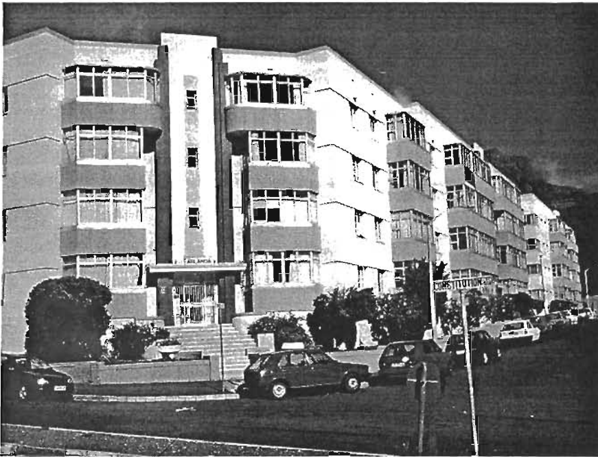
Figure 6.6 The Bloemhof Flats (The enclosure and plastering of the balconies is a recent change)
