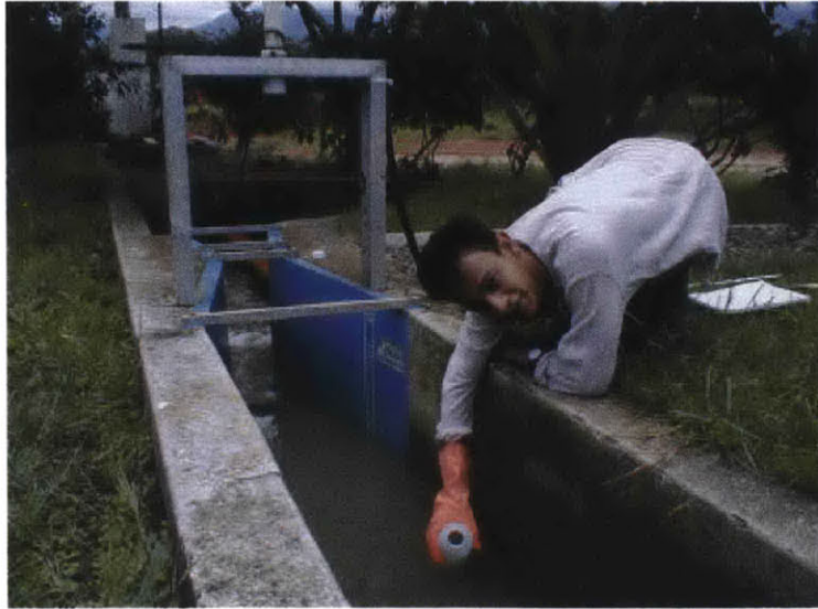
Figure 27: Sampling Point E-6, Final Effluent – From Chlorination Tank
