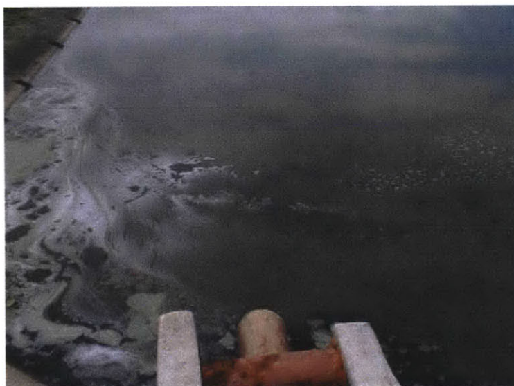
Figure 28: Floating 'Sludge Bombs' in the Facultative Lagoons
