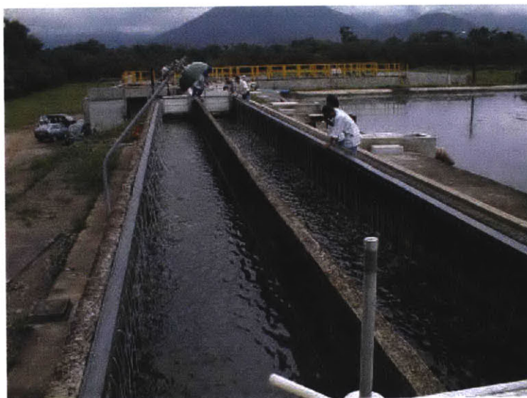
Figure 9: Flocculation Chambers (23m long)
