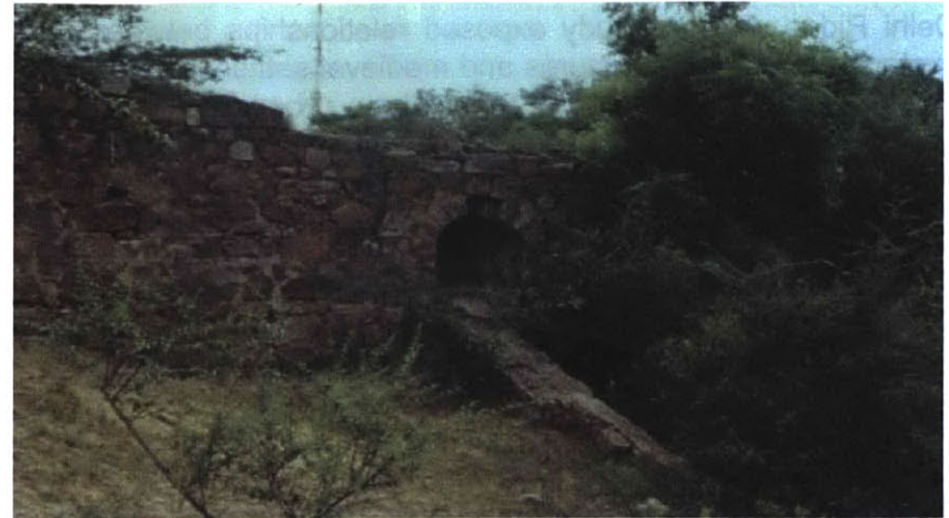
FIG. 2-7. The Bundh at Dasghara Village, as viewed from the erstwhile reservoir. The typical ' mori ' (round apertures) opening could be variably opened.
