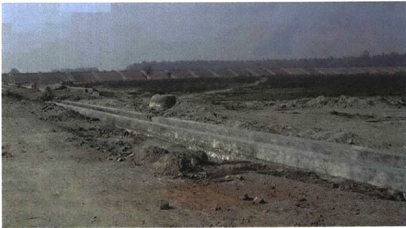
FIG. 1-6. Drains and Embankments to Protect the CWG Village Site.
