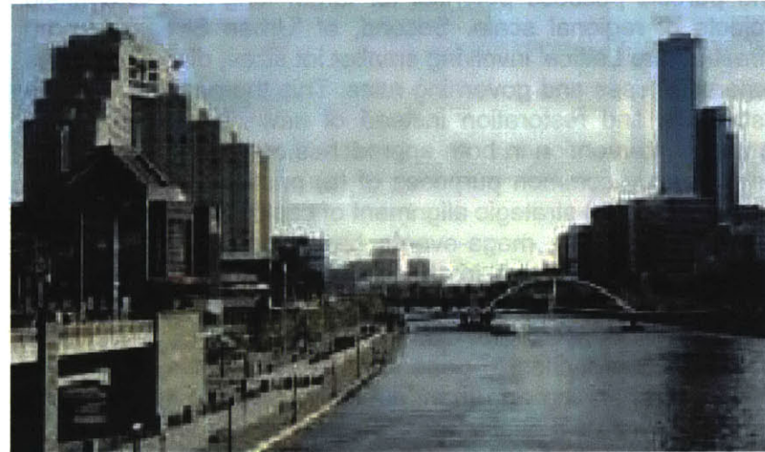
FIG. 4-1. Waterfront Development along Yarra River, Melbourne. Preparations for the CWG 2006 have been focused along the ‘leisure corridor’ along the river’s stretch through downtown.
