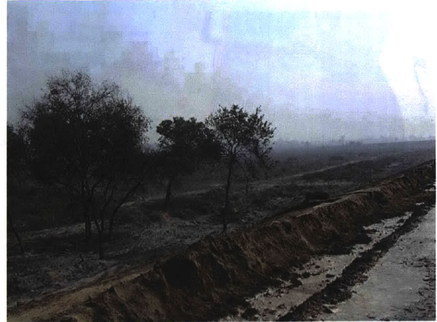
FIG. 1-5. Earth Piled Atop Flood Embankment along the CWG Village Site. The sandy, flood-prone soils cannot sustain most tree species. Note the withered plantation.
