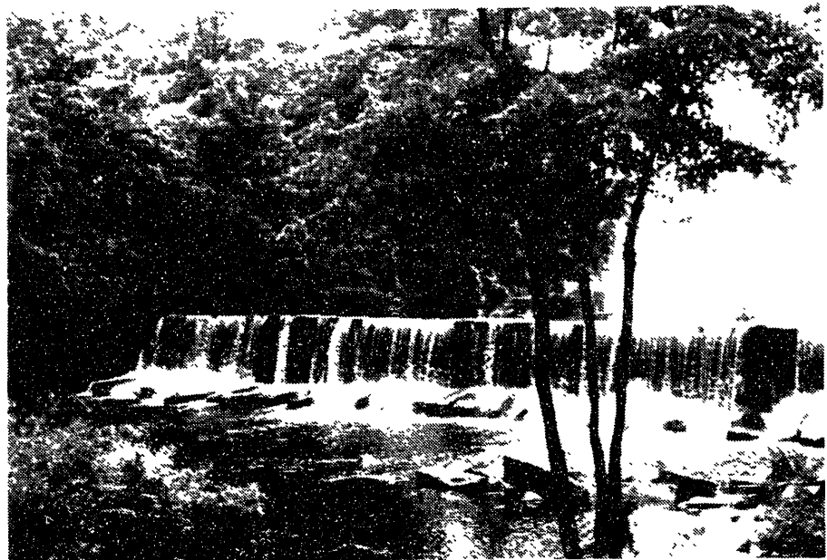
Fig. 2-5. Dam at Townsend Harbor mill site on the Squannacook.
