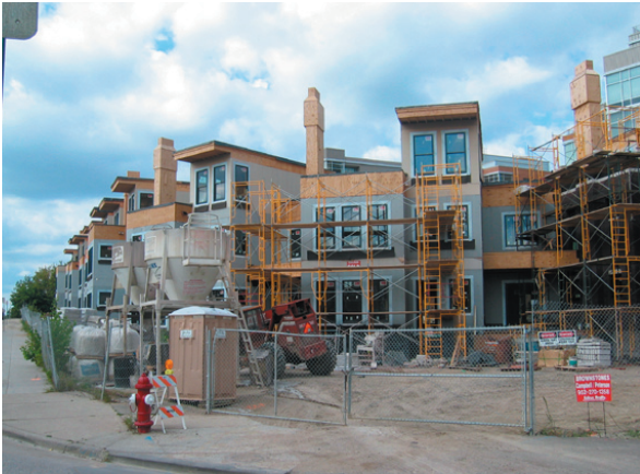
Condominium development on Northeast Minneapolis riverfront.
