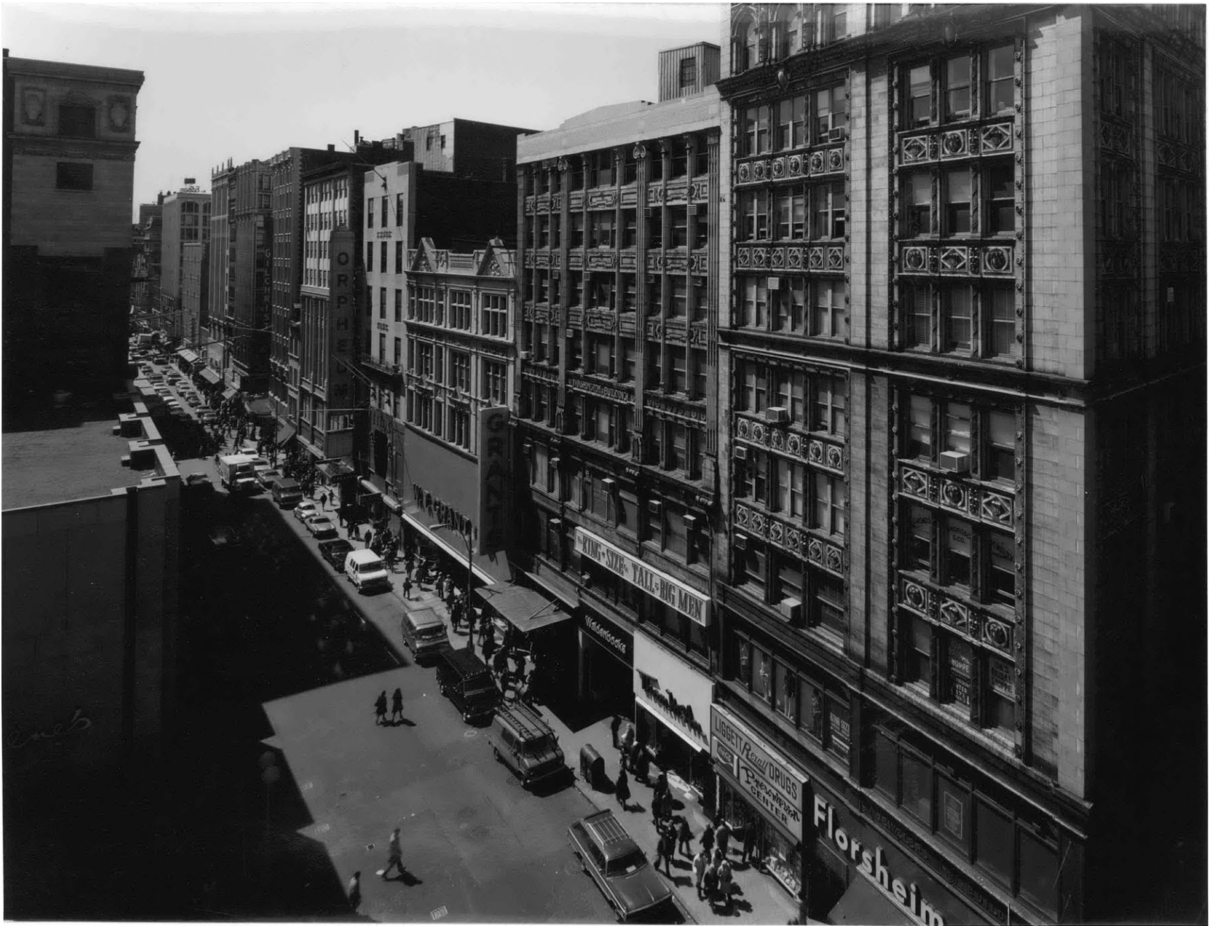
Fig. 42 West side, looking south from Bromfield Street 1976
