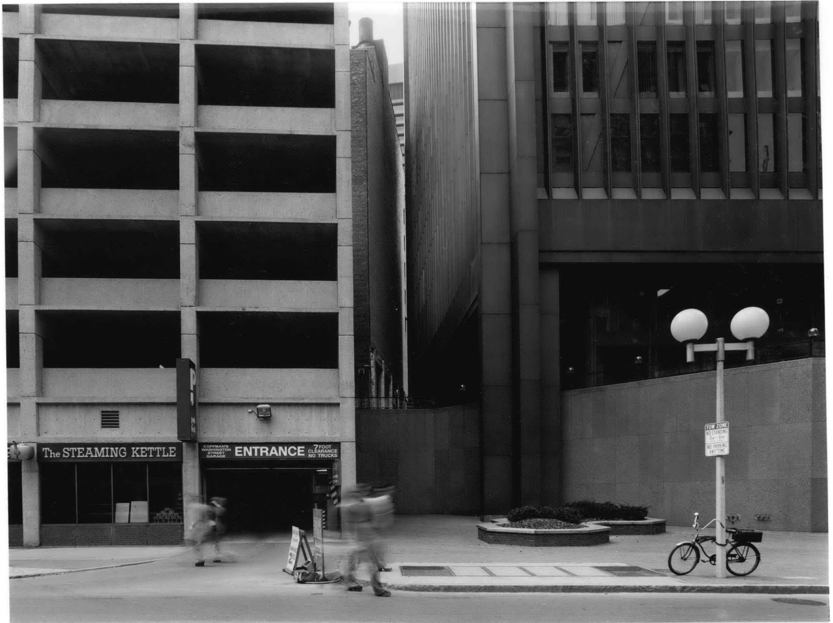
Fig. 71 Pi Alley Cinema and the Boston Company Building 1976
