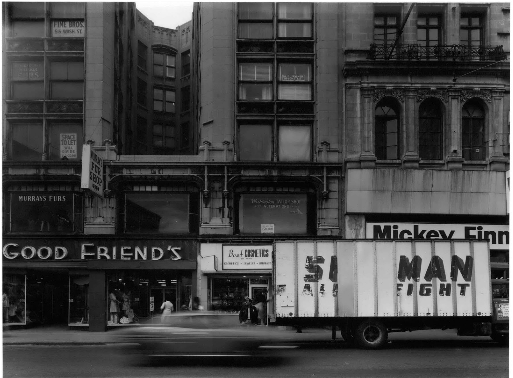
Fig. 11 West side of Washington Street near West Street 1976
