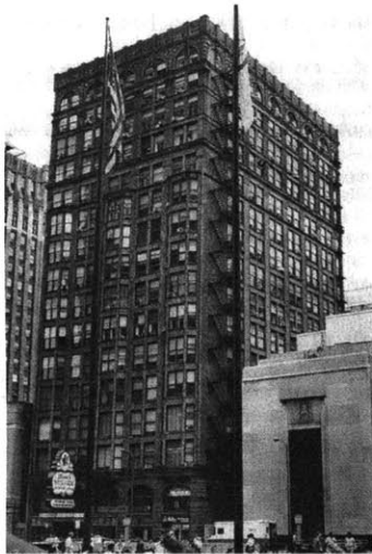
FIG. 8.4. Unity Building with ComEd substation on right.
