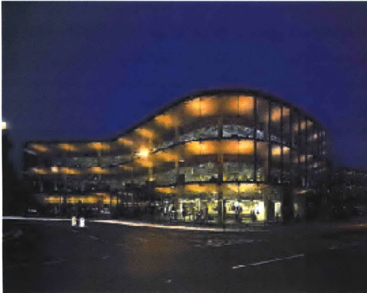
FIG. 2.8. Willis Faber and Dumas Building, Ipswich, England. Foster and Partners.
