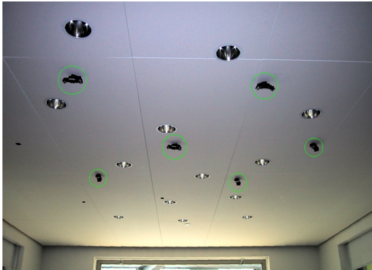
Figure 3-2: Beacons are generally placed on the ceiling to provide coverage throughout the room. In this photograph, the Cricket beacons are circled in green.
