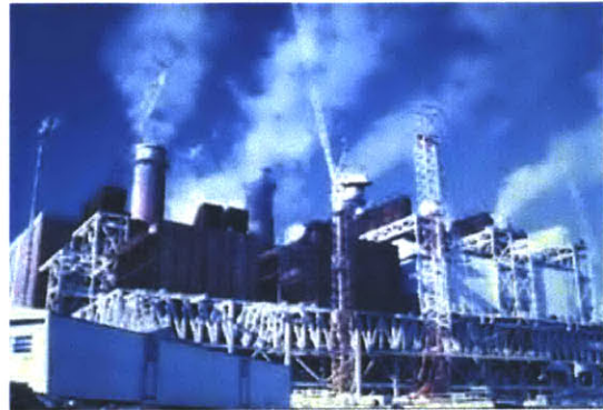
Figure 2.1: Electricity plants produce over 70% of air pollution
