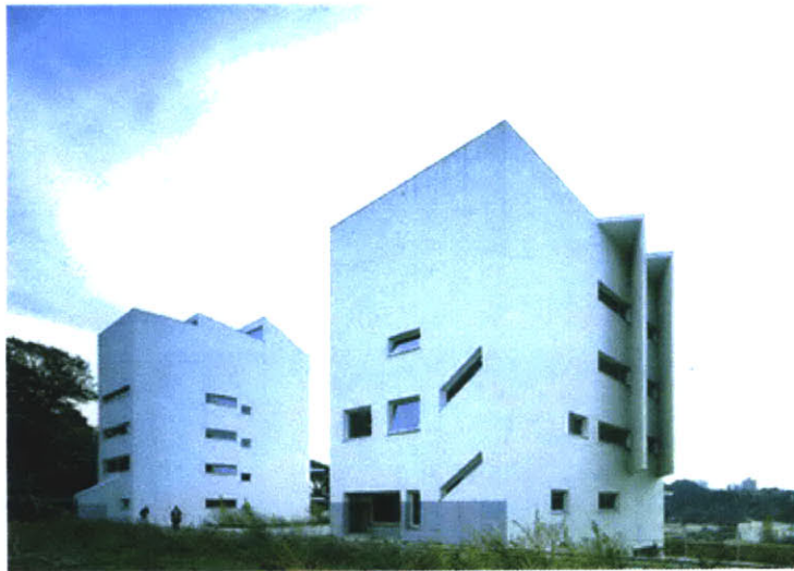
Figure 7.3 Northwest view of towers H and G. Tower H is in the background. Tower G is in the foreground, showing the large vertical fins that protect the west-facing studio windows from direct sun.
