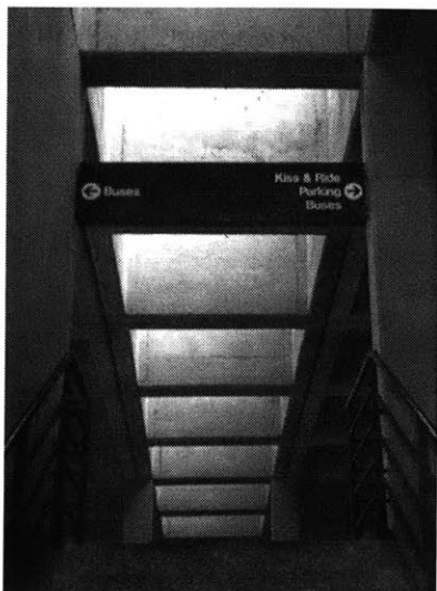
Figure 4.42 West Falls Church/VT-UVA Station Fairfax County, Virginia
