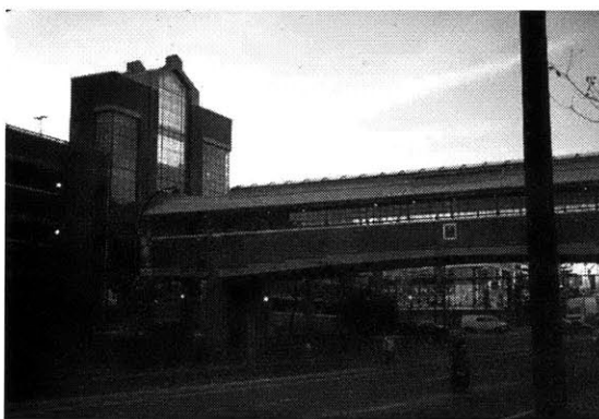
Figure 4.5 Pedestrian bridge over Viers Mill Road with parking garage at left; Metro entrance (not seen) at right
