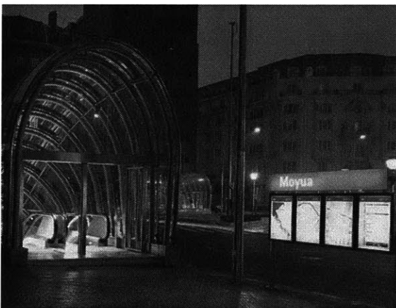
Figure 4.45 Moyua Station Bilbao, Spain
