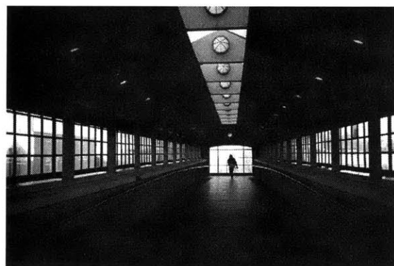
Figure 4.6 Interior of the pedestrian bridge with architectural detailing
