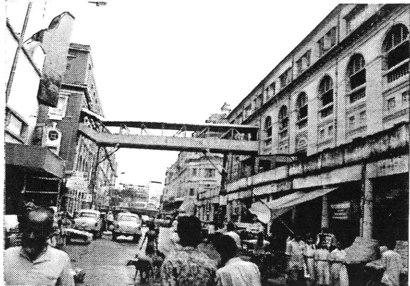
Overhead access between Corporation Building and arcade on Hogg Street.
