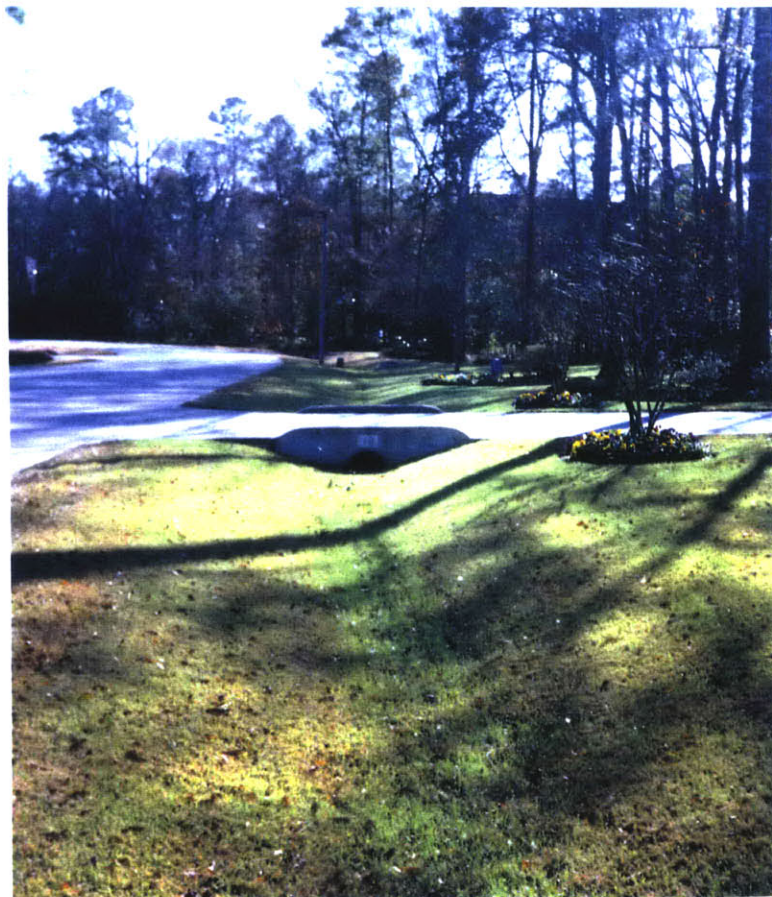
Figure 5. Drainage in The Woodlands. Top photograph is of typical grassed channel that has replaced naturally vegetated swales proposed by WMRT. Lower photograph (taken off Watertree Drive) is of grassed stormwater swale on residential lots in the estate section of Grogan's Mill. The type of drainage depicted in the lower photograph is largely restricted to Grogan's Mill.
