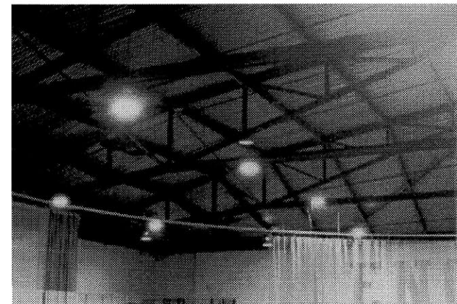
Roof trusses, W34, Johnson Athletic Center
