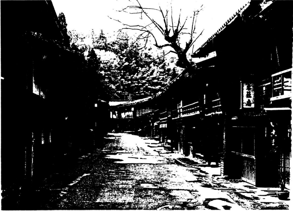
Figure 36: View south to Terashita
