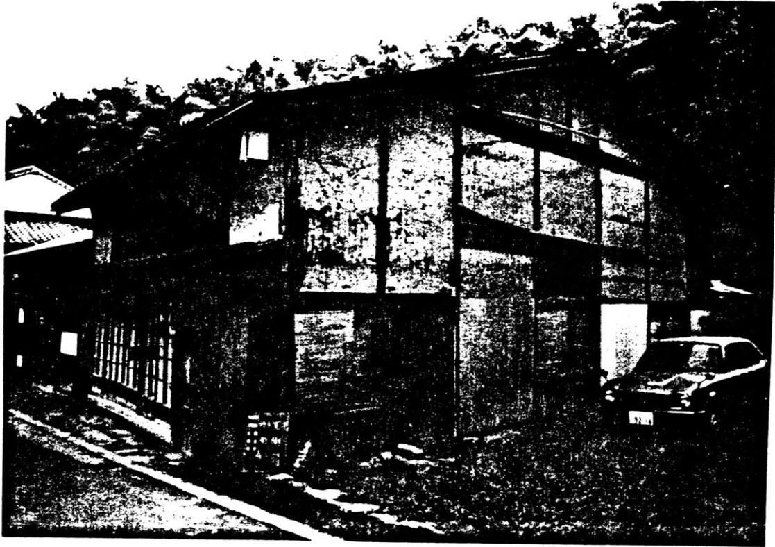
House in Nakamachi before restoration
