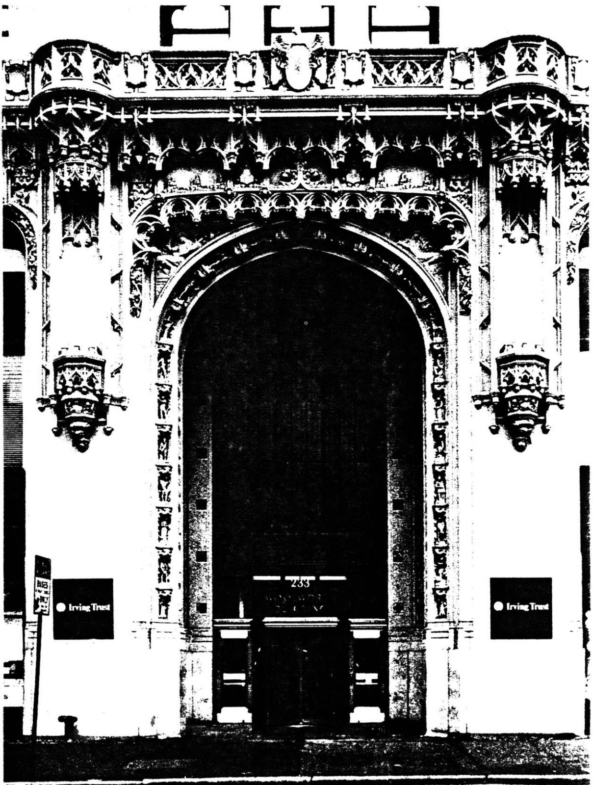
259. Woolworth Building, main entrance
