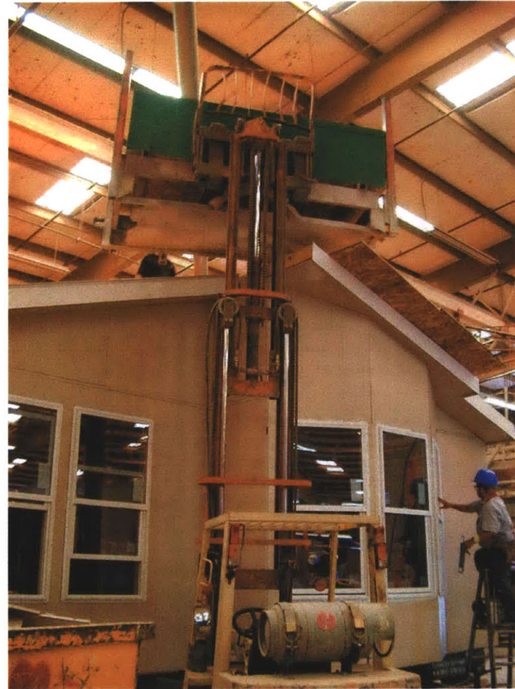
The Corona, CA factory of Silvercrest Western Homes operates an efficient and safe business. They point to quality control and financing advantages as the reasons for their success.
