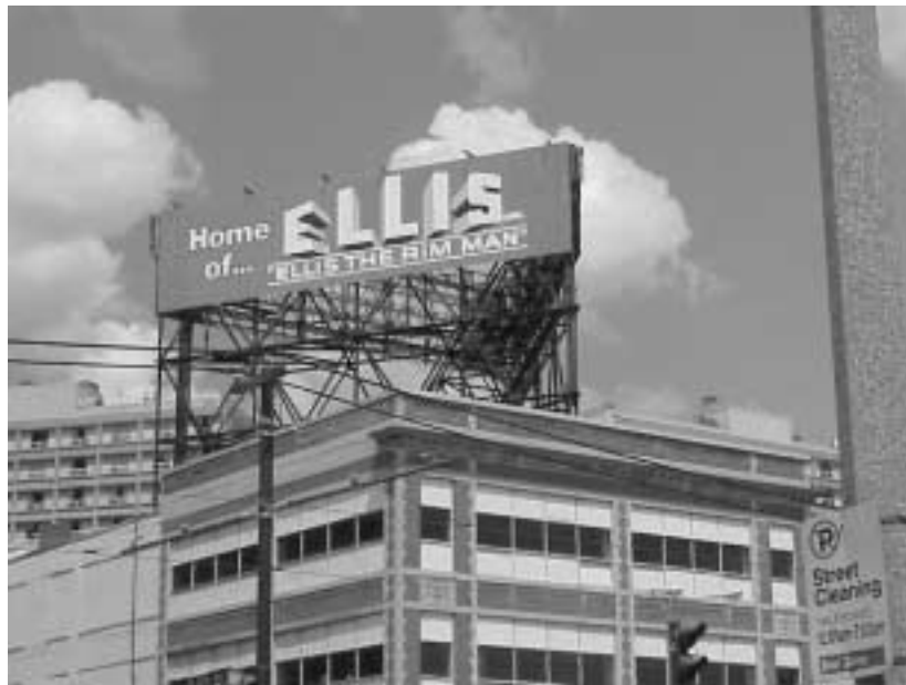
Figure 5.6 This billboard on Commonwealth Ave. utilizes triangular truss elements.
