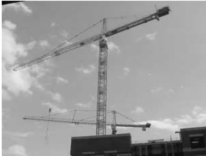
Figure 5.1 Construction cranes near Haymarket in Boston make use of truss structures.
