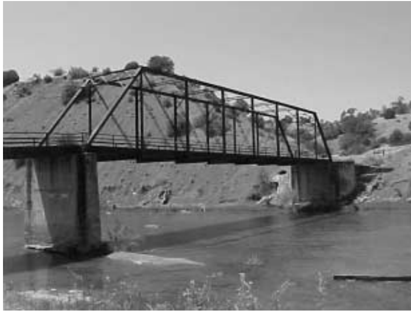
Figure 5.4 A truss bridge in Glenn County, CA. [Taken from Truss Bridges of Northern California : http://community-2.webtv.net/DAROSAMAR-CIELII/TrussBridgesOf , October 2001.]
