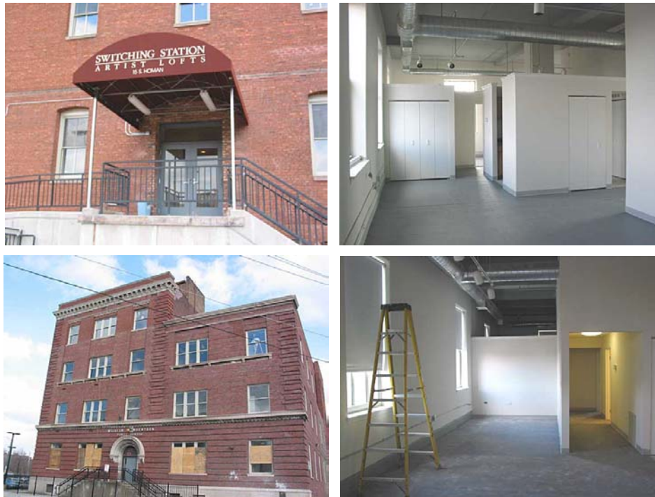
Figure 4.6 The exterior and interior of the new artist live/work housing
