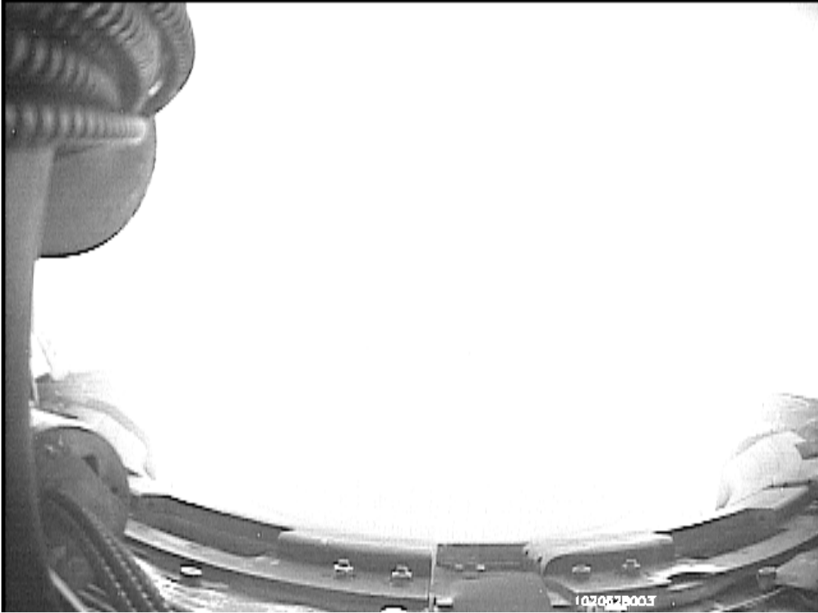
Figure 4-56: “F-port” Wide-angle view image taken before the viewing dump (in the near field) is bent. In this image the cabling on the left side of the view is clearly visible.
