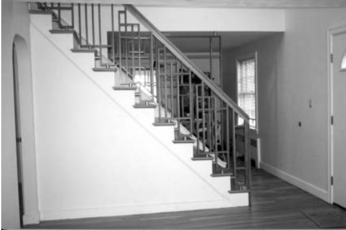
Figure 8.27: Screenifying the stair: a wall has been replaced with a screen in the Chatham house.
