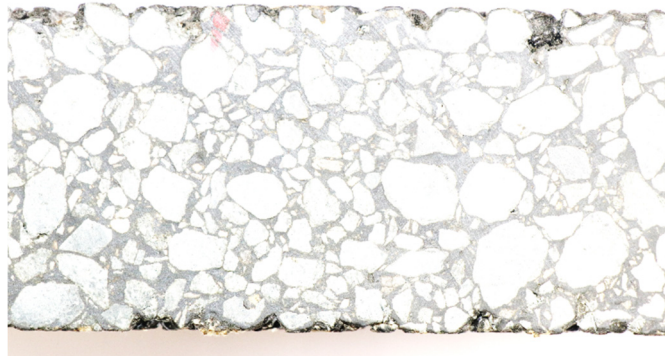
(b) Surface condition of ASP specimen
