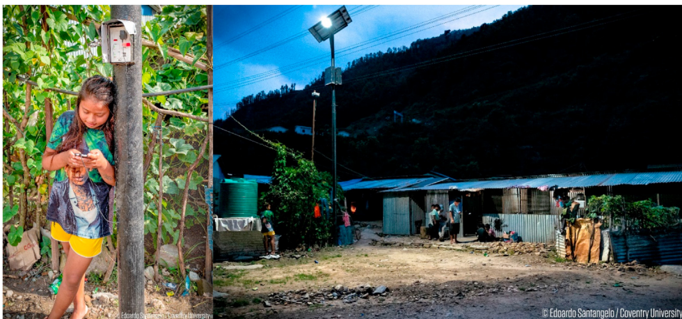
Fig. 9. A solar streetlight in Uttargaya, Nepal, being used to charge a phone and provide lighting at night.
