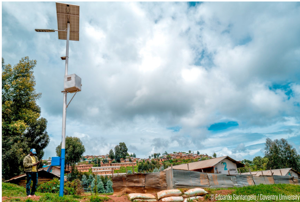
Fig. 5. An advanced solar streetlight with sockets installed at the entrance to Gihembe refugee camp, Rwanda.
