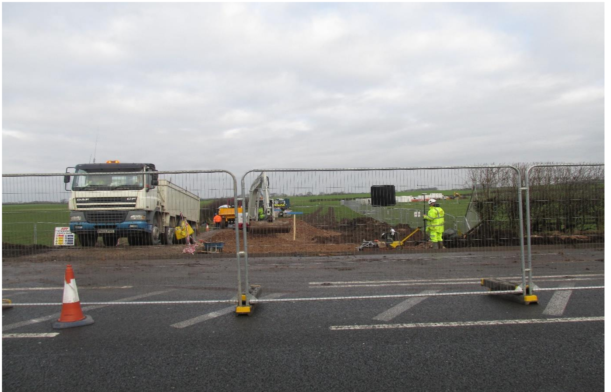
Figure 5.28: Picture of work in progress at Preston New Road drilling site
