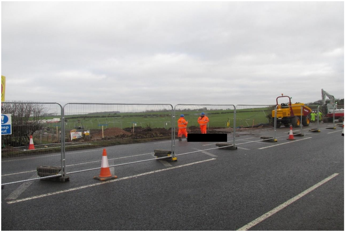
Figure 5.26: Preston New Road drilling site with work on-going
