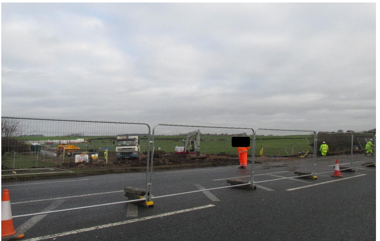
Figure 5.29: Overview of Preston New Road drilling site
