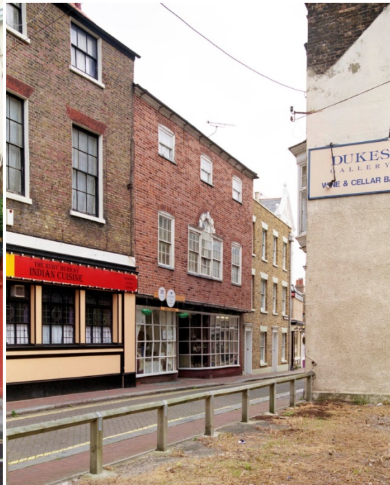
Fig 9 Refronted timber-framed house in Duke Street, Margate [AA050566]
