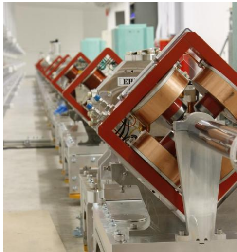
FIGURE B.2: Picture of a quadrupole magnet in the tunnel of the TRIUMF linac. From [152].
