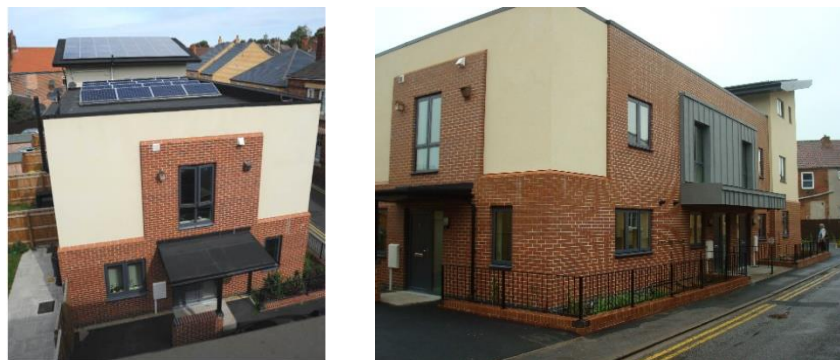
285 286 Figure 1 . UK houses Gainsborough (a) south elevation, UK_H1 in foreground; b) east elevation 287
