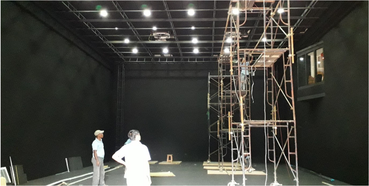
Fig. 3: MMPDD Film Centre, Studio 1 refurbishment.
