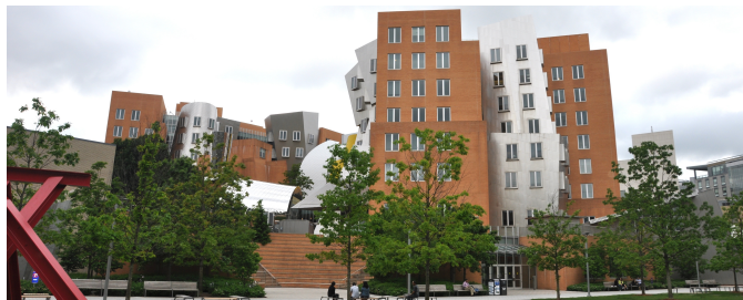
Fig. 1. Ray and Maria Stata Center designed by Frank O. Gehry and completed in 2004. The 10 floor, 67,000 m 2 building is the home to the Computer Science and Artificial Intelligence Laboratory.
