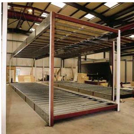
(a) A typical primary steel frame
