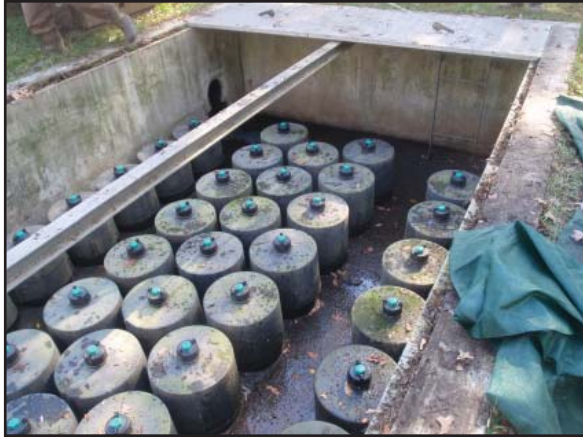
Figure 1: ZPG cartridges in filter system.
